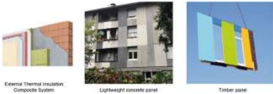
Fig. 2 The three different technological solutions
