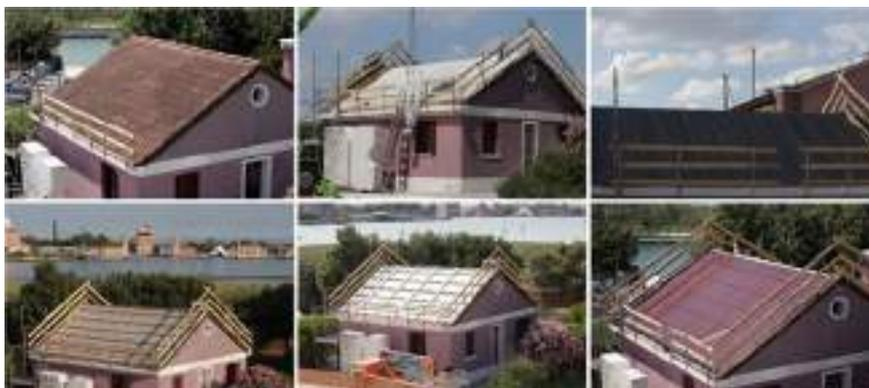
**Fig. 3** Construction phases of a BIPV roof. *Source* GruppoSTG/VDV srl
